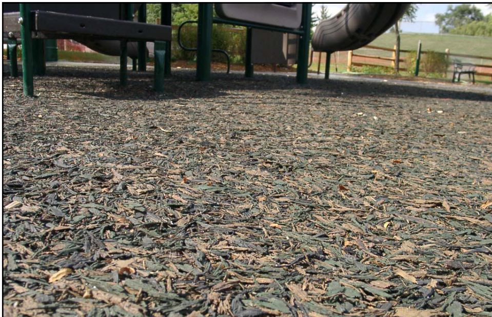
Large piece shredded rubber is mixed with a binding product to make a unitary surface.
