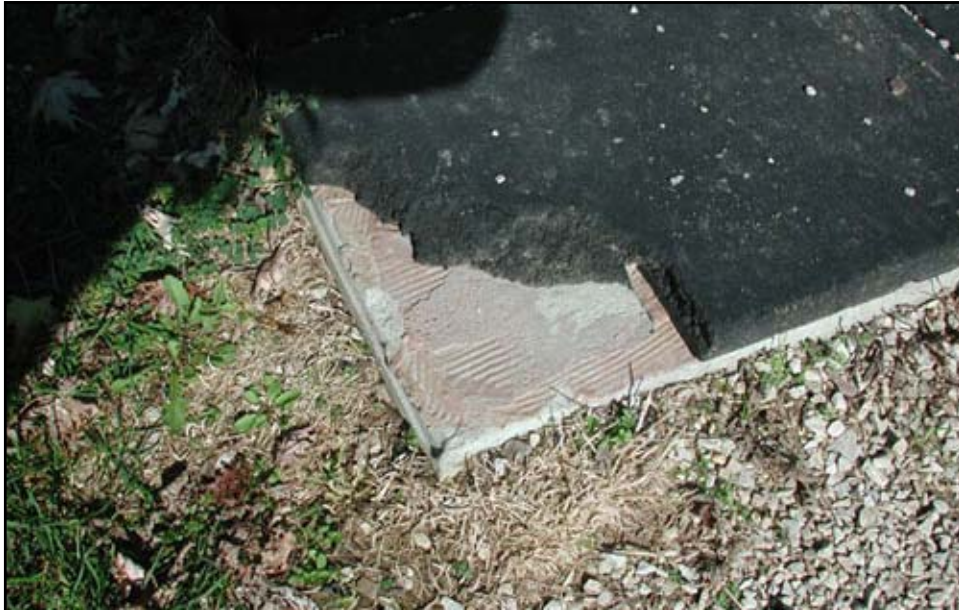
The corner of the rubber tile has broken away to expose the concrete base.
