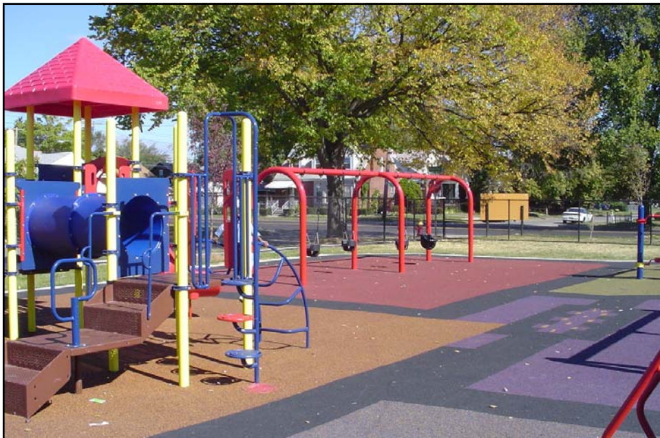
Poured in place rubber surface system in multiple colors, leads to composite structure and swing bays. From the City of Detroit.
