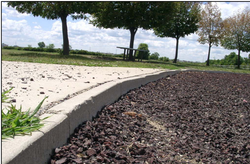
A concrete walkway and curbed containment border lead to a loose fill playground surface. There is a 6-12" drop from the concrete into the loose fill.
