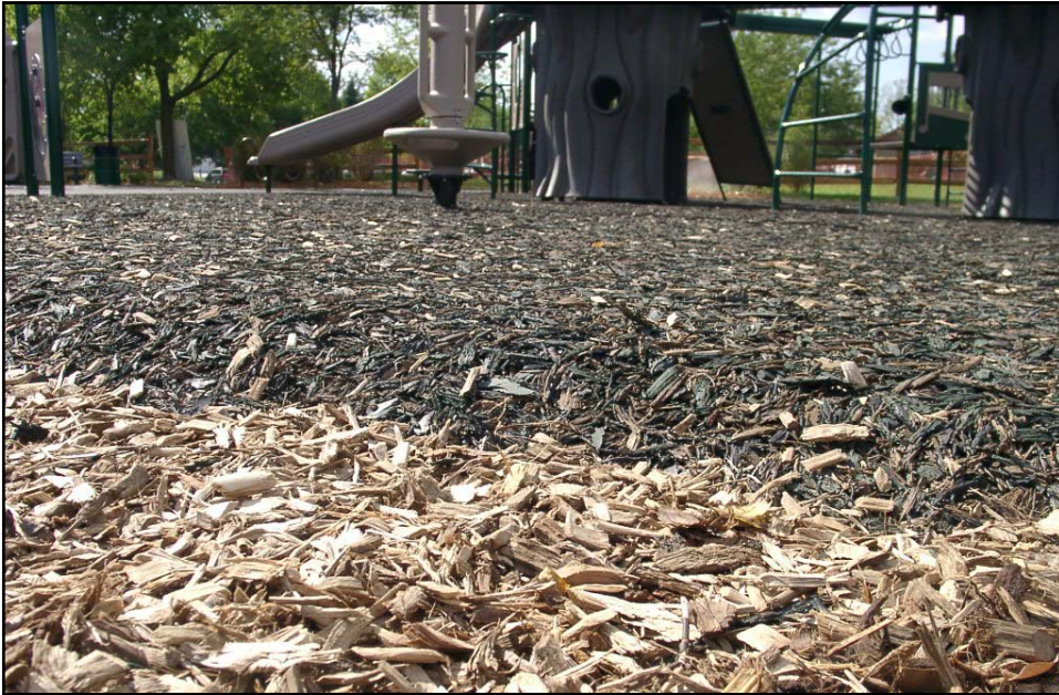
The large piece bound shredded rubber has a beveled transition meeting with loose fill wood product.
