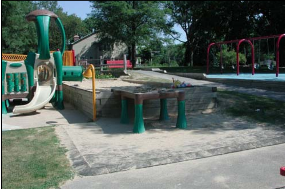
Raised sand area built into landscape and contained by wood timbers with adjacent sand table. Crawl tube from elevated play structure empties into raised sand bed.
