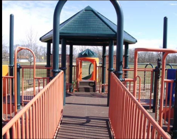
Right: An elevated platform wide enough for wheelchair passage connects the same two platforms of the elevated composite structure.
