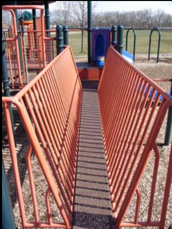
Left: An elevated balance beam with side barriers connects two platforms of an elevated composite structure.
